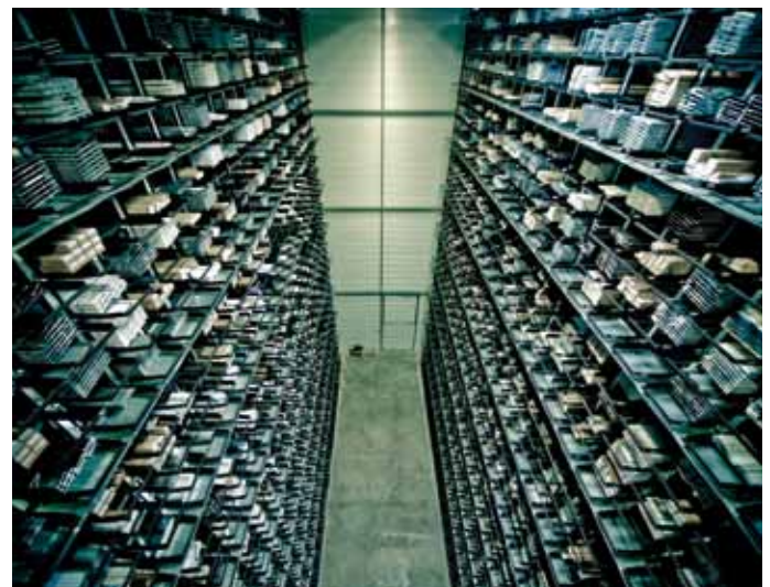
Installed in 2009, with more than 1800 storing places, the second High-Storage Automated System of GUTMANN in Weissenburg.
