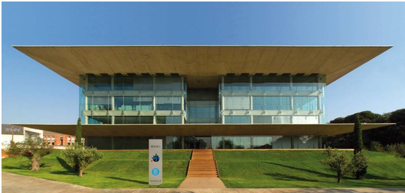
NEXUS OFFICE BUILDING. BARCELONA
